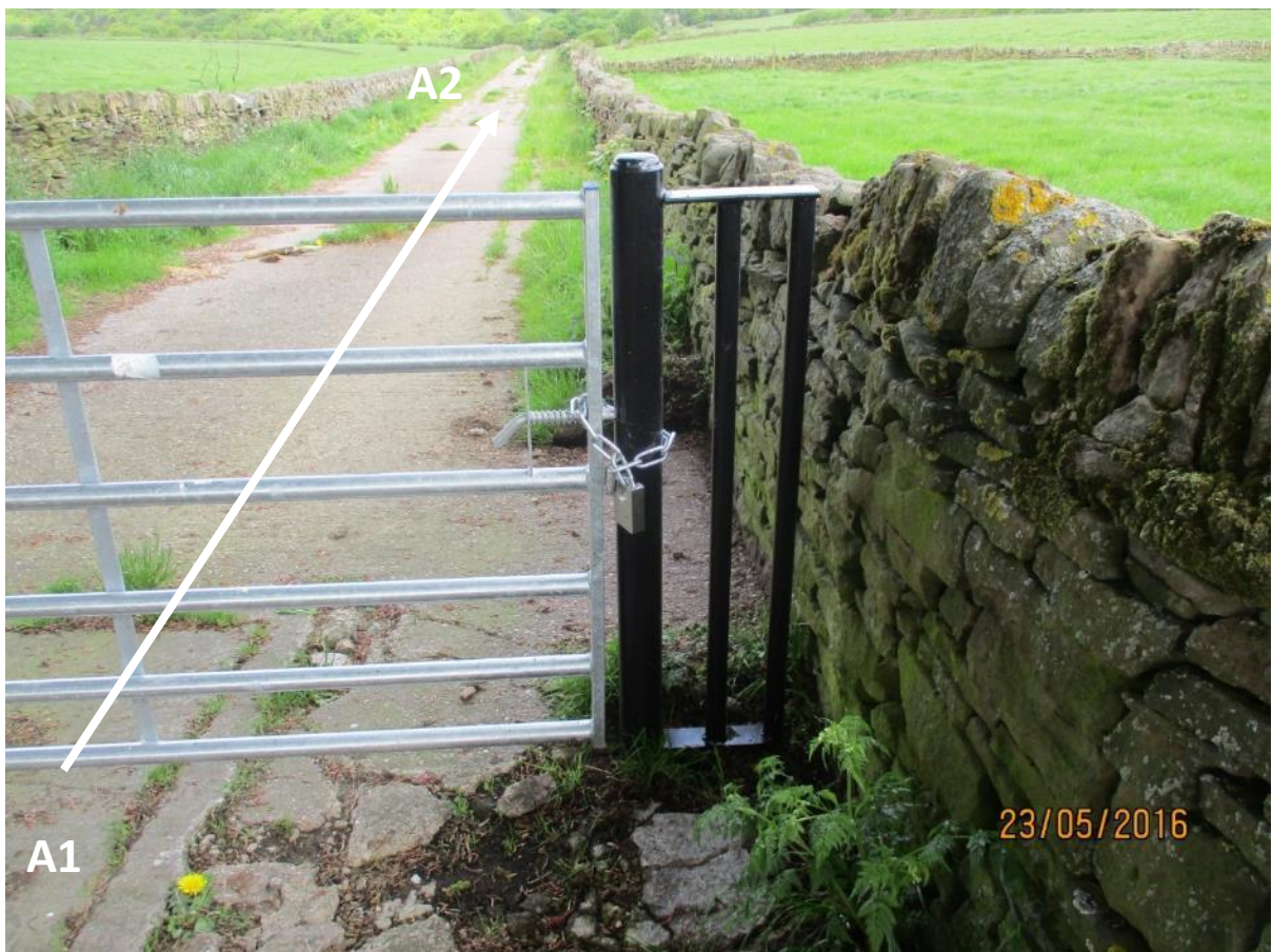
12. Padlock and chain on new gate at A1. 23 May 2016.
